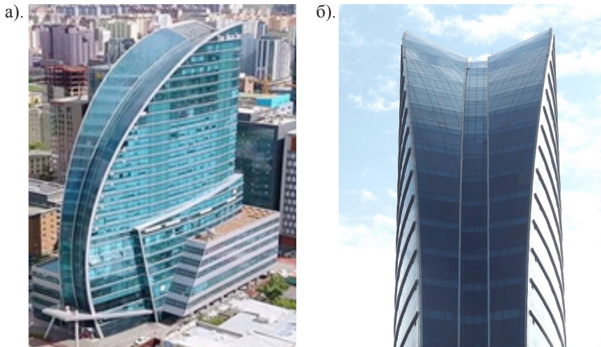
Fig. 9 – Hotel "Blue Sky": a - general view; b - roof shape
