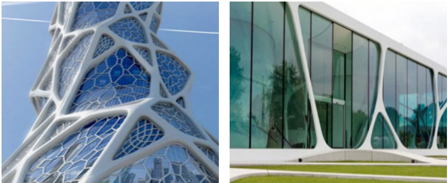
Fig. 2 –Examples of bionic style in modern buildings
